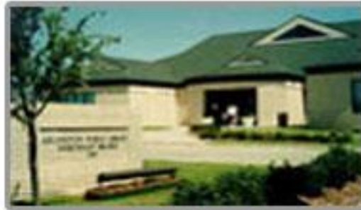
Northeast Branch Library
